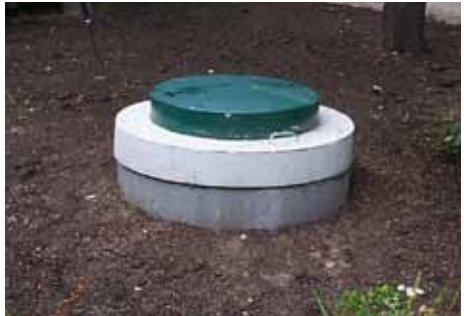
Photo courtesy of Simon Smith Drilling Ltd.
