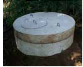
Photo courtesy of Simon Smith Drilling Ltd.
